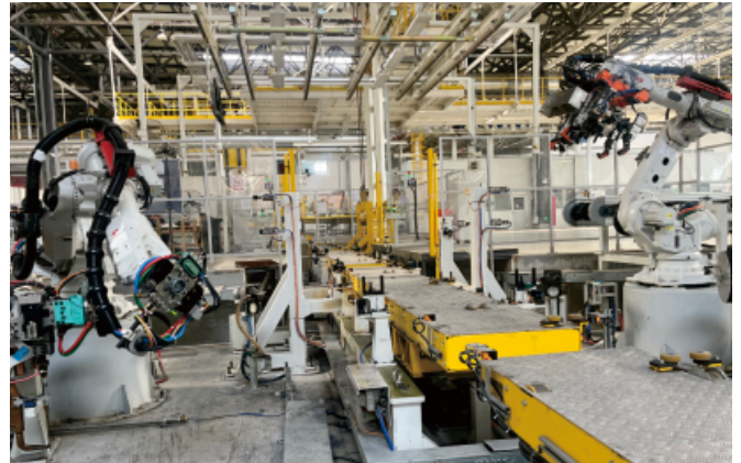
Body welding main line
